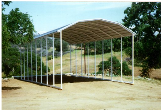
Carport structure similar to ours.
